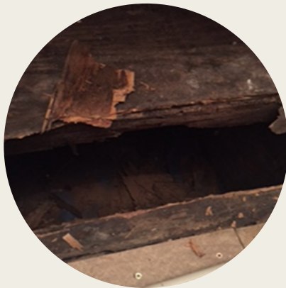
A timber floorboard and joist damaged by wet rot caused by a water leak over a long period of time.
