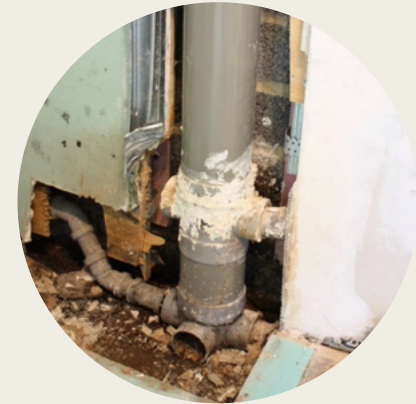
A soil stack carrying foul water from toilets and baths located within a block of flats, running from top to bottom of the block.
